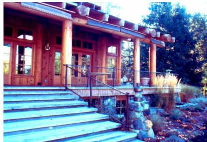
Fig. 14. Brown Lodge Porch Detail.
